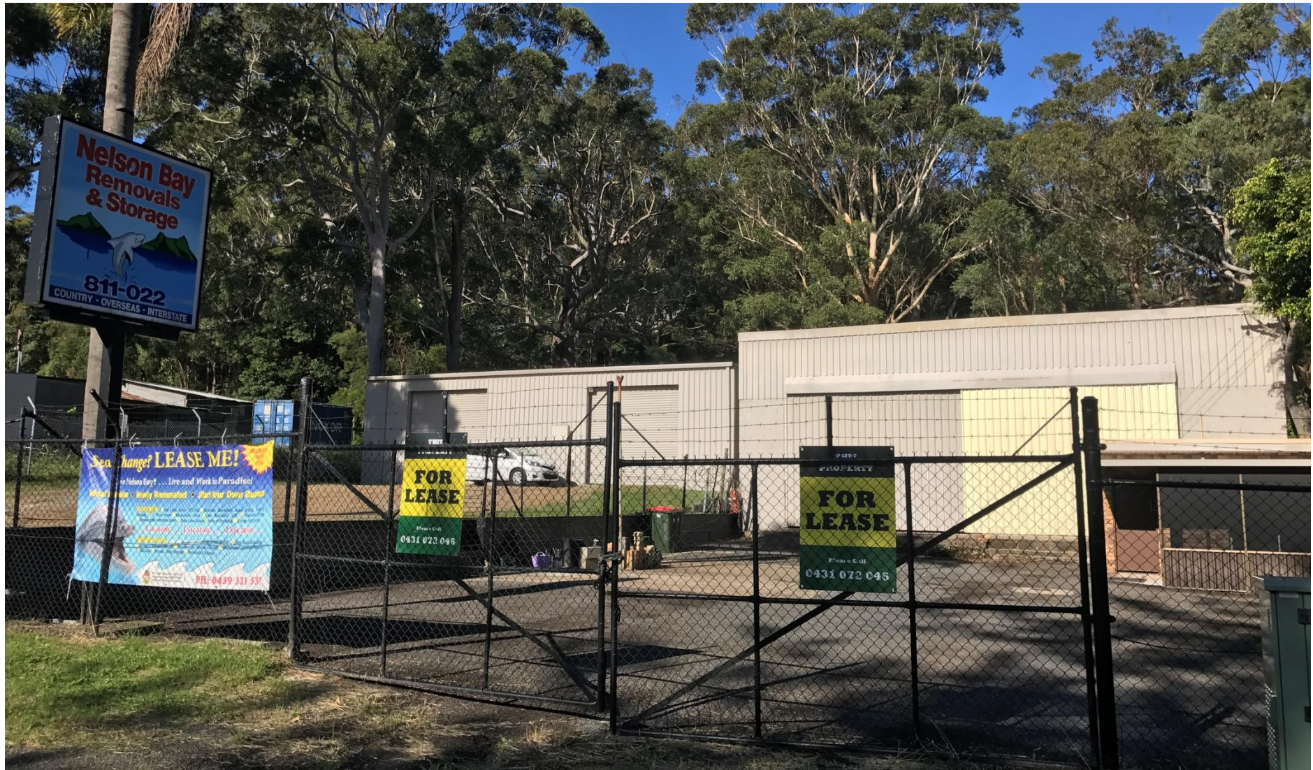
Figure 4: Existing structures at 95A & 97 Stockton Street, Nelson Bay
